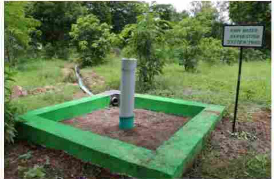
Roof top Rain Water Harvesting System at plant
