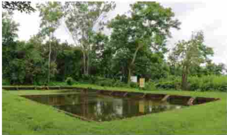
Surface Rain Water Harvesting System at colony
