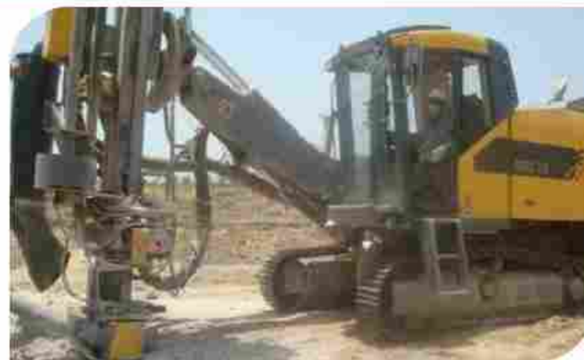
USE OF PPEs BY DRILL OPERATOR
