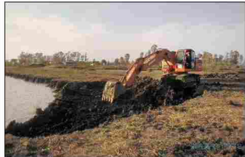
Pond Deepening work for Water Harvesting at Futera Pond, Damoh
