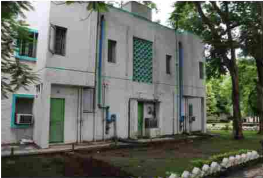
Roof top Rain Water Harvesting System at plant
