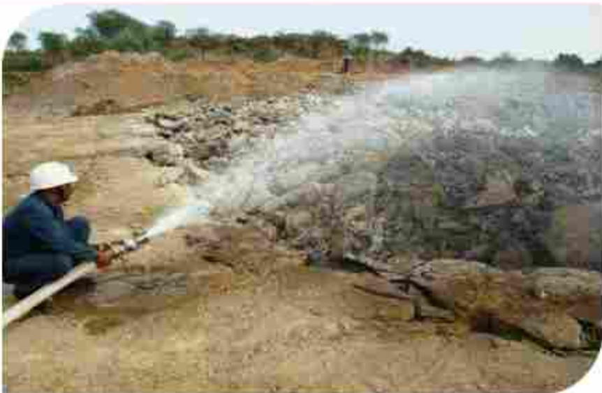
WATER SPRINKLING ON BLASTED MUCK
