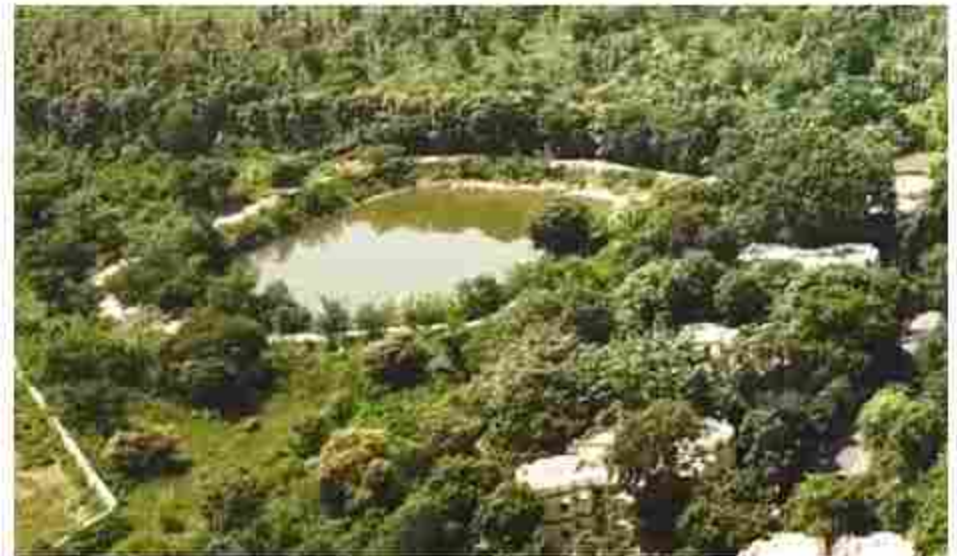
Water Reservoir at plant Colony
