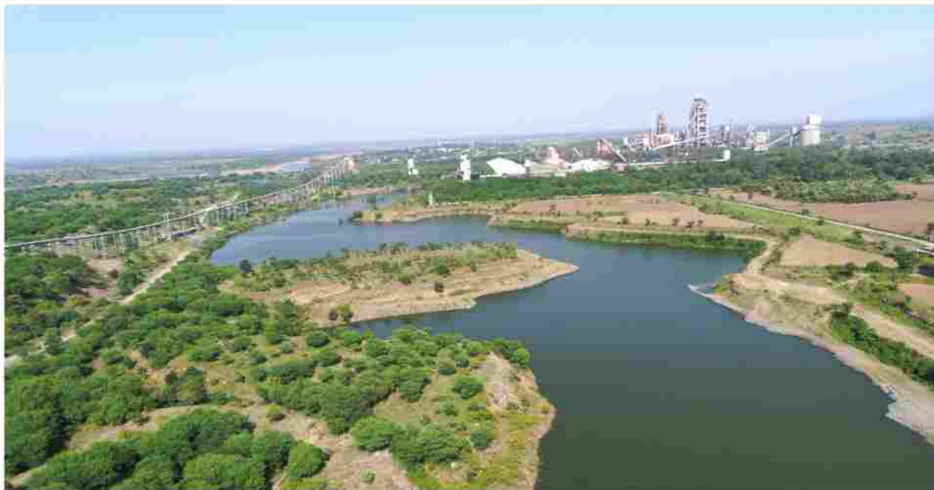
Water Reservoir Narsingarh Village
