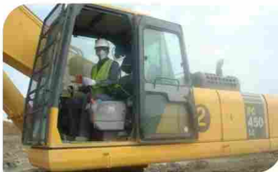
USE OF PPEs BY EXCAVATOR OPERATOR HEIDELBERGCEMENT
